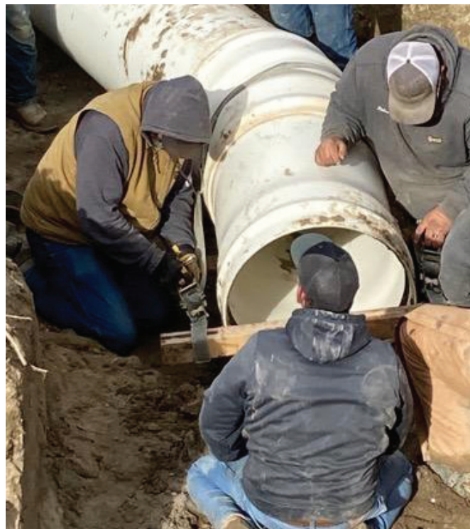
Using tiedown straps and ratches to seat the pipe into the elbow.
