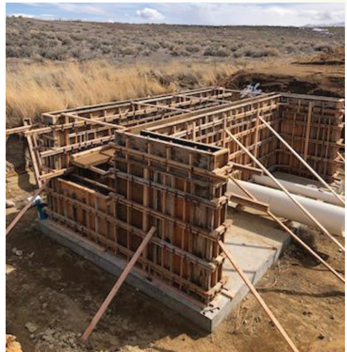
Turnout construction in the main canal.
